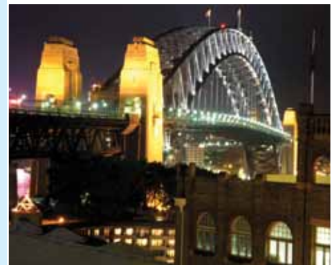
Sydney Harbour Bridge
